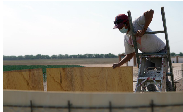
Photo: A community member in the process of building a Rainwater Harvesting System. In the background, a section of a modern agricultural field is visible, with a private well and irrigation systems, in a region of extreme water scarcity.
